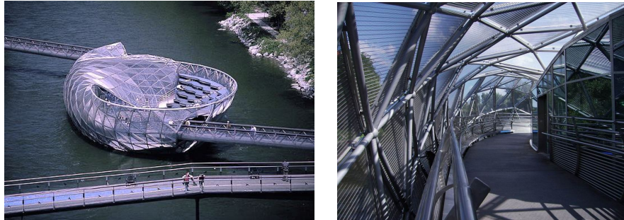
Figure 03 Triangulation, Murinsel Graz
