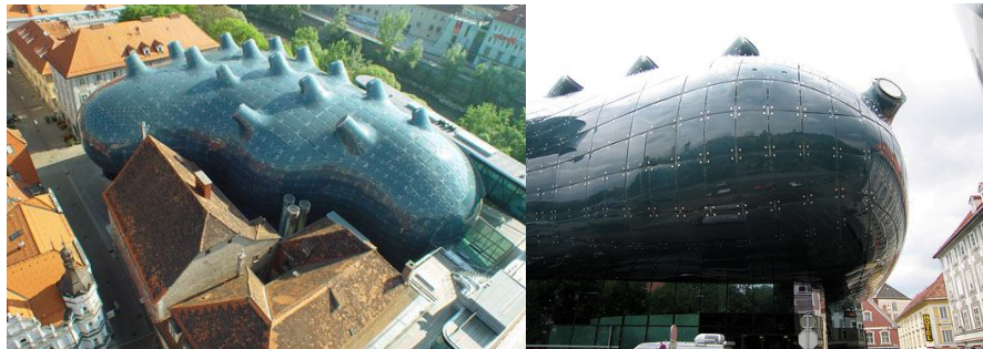
Figure 01 Discretization with curved segments, Kunsthaus Graz
